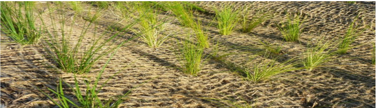
Installation of Jute Geotextiles on Slopes for Industrial Site Development
