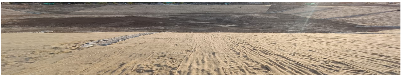
Ocean Jute Geotextiles Installed for Slope Stabilization in Waterpond Project
