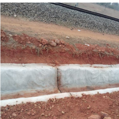
Ocean Gccm Applied in Mountain Terrains for Drainage Purpose (Project 1)
