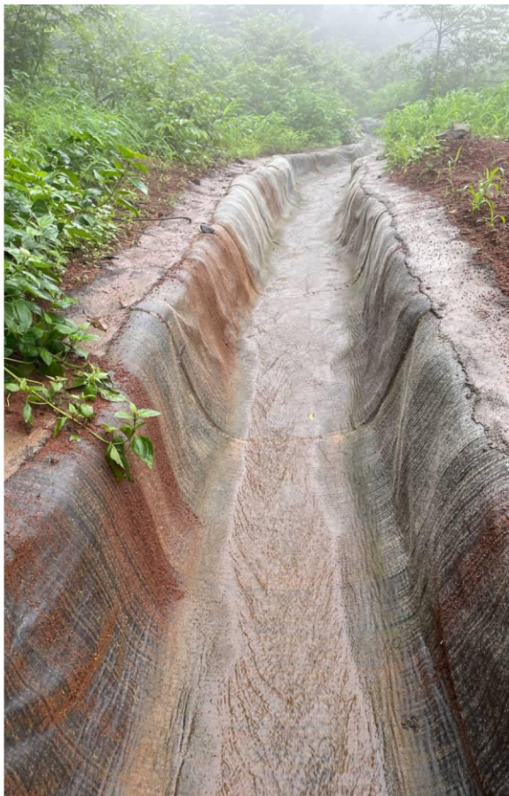
Ocean Gccm Applied in Mountain Terrains for Drainage Purpose (Project 2)
