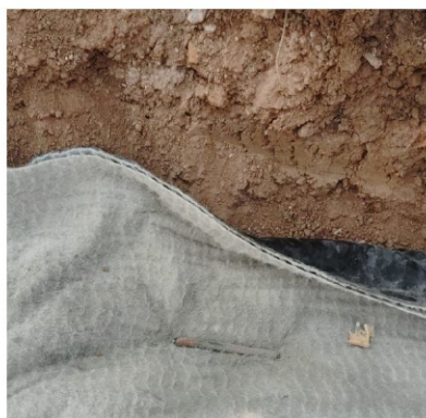
Ocean Gccm Applied in Mountain Terrains for Drainage Purpose (Project 1)
