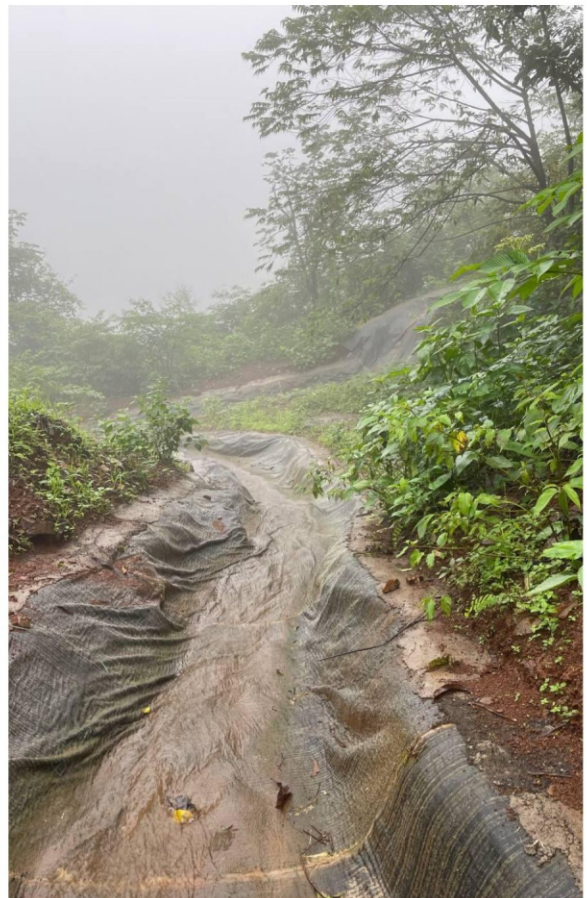
Ocean Gccm Applied in Mountain Terrains for Drainage Purpose (Project 2)
