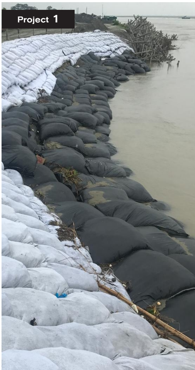
Installation of Ocean Geobags for flood fighting at Brahmaputra river-front project, Assam
