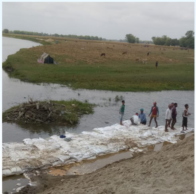
Ocean Geobags installed for riverbank protection, Bihar
