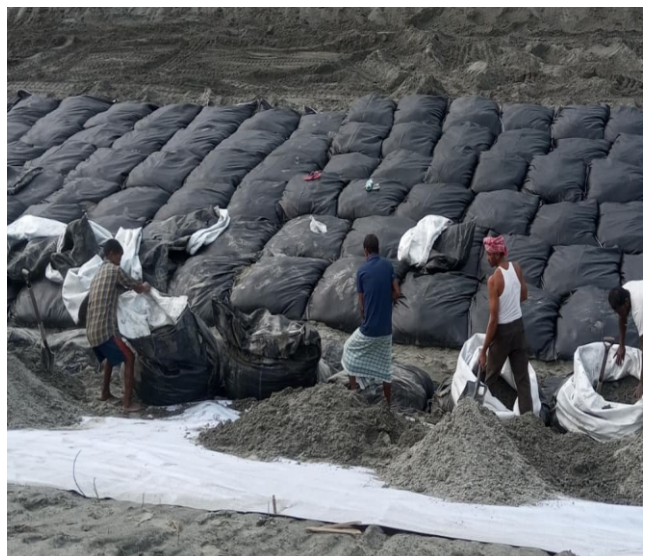
Installation of Ocean Geobags for flood fighting at Brahmaputra river-front project, Assam
