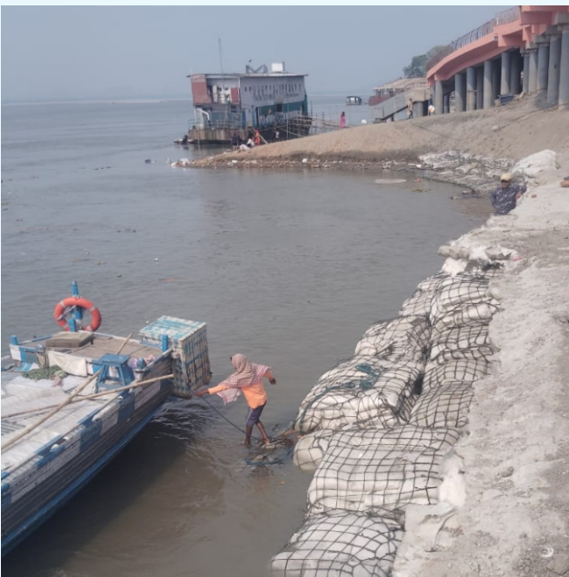
Ocean Geobags installed for riverbank protection, Bihar
