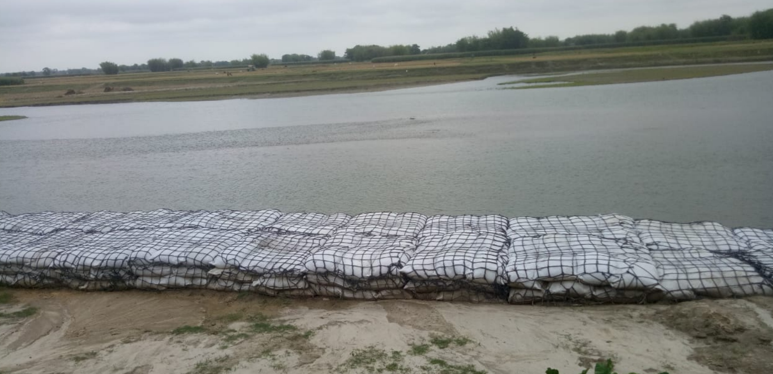
Ocean Geobags installed for riverbank protection, Bihar
