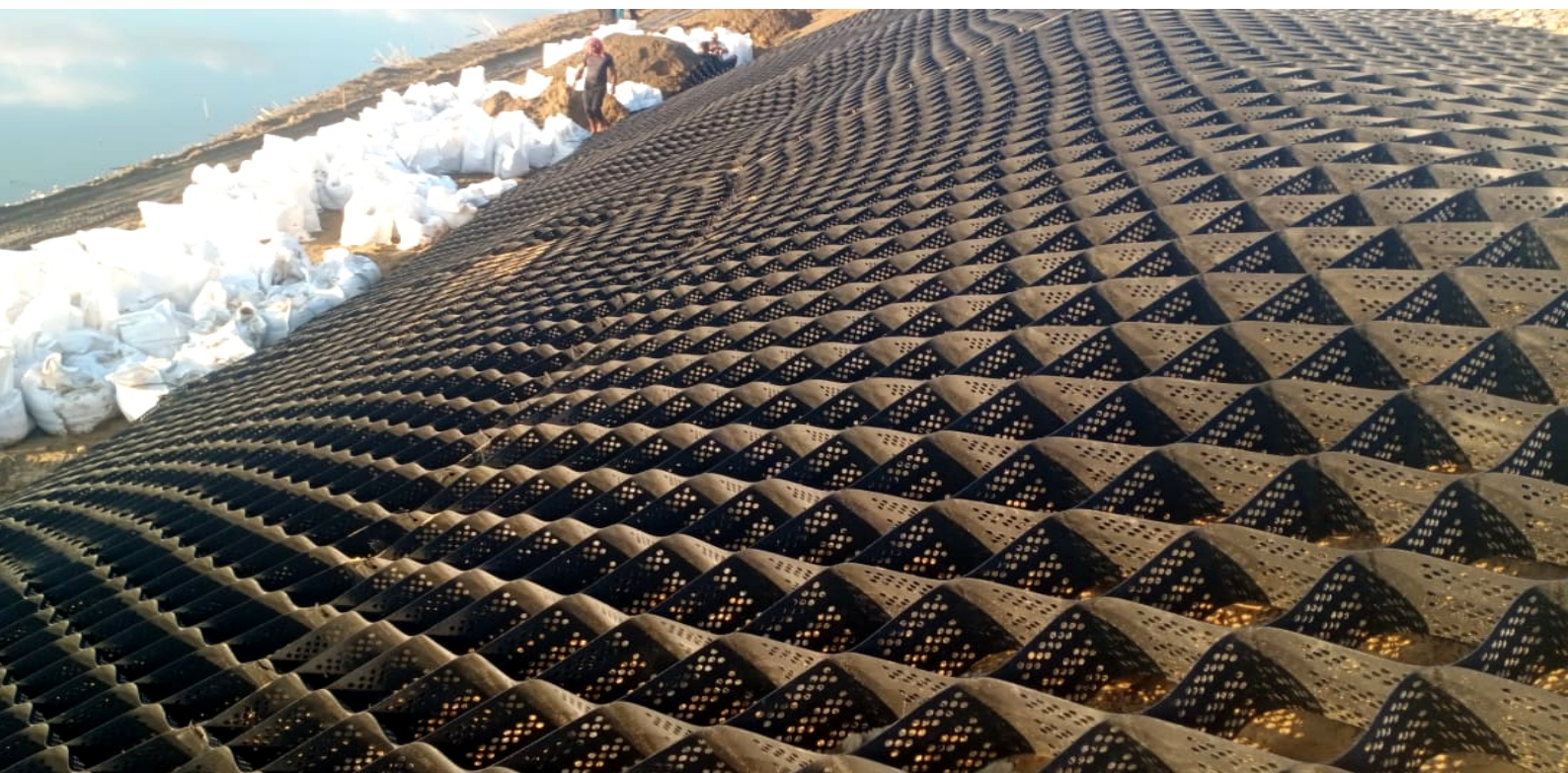
Geocells for slope embankment for a railway project.
