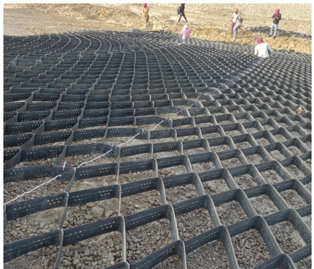
Geocells for slope protection for NHAI project.
