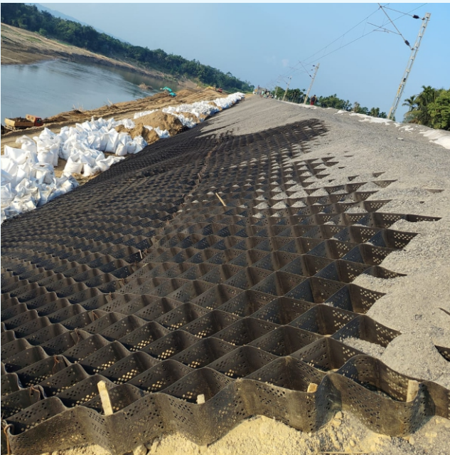
Geocells for slope embankment for a railway project.
