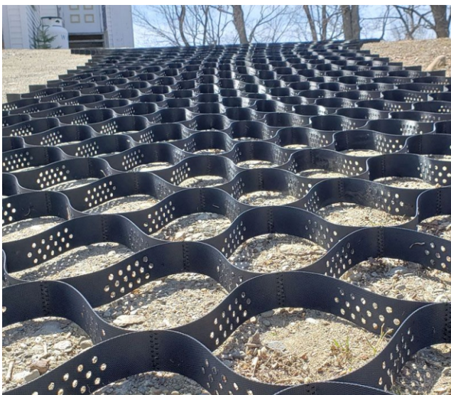
Geocells for slope protection for NHAI project.
