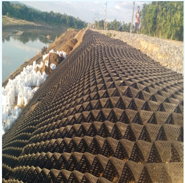
Geocells for slope embankment for a railway project.
