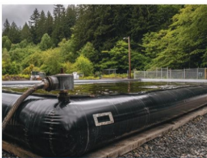
Geo Tube Dewatering Containers
